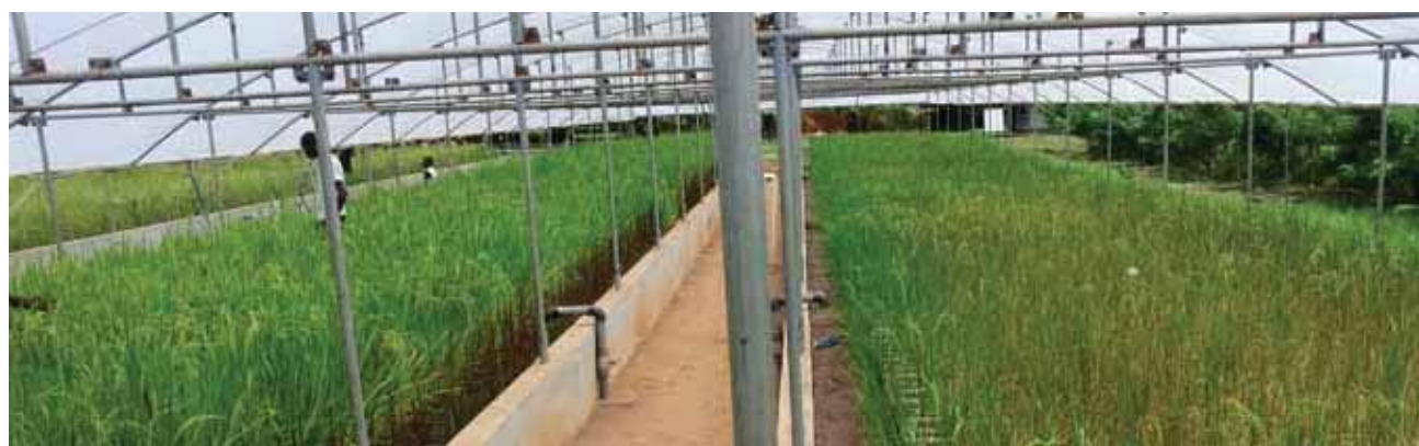
The controlled lowland-drought facility at AfricaRice headquarters in Cotonou consists of four rainout shelters, each 5 m × 68 m. The traits being measured include visual scores, phenology, yield, yield components, leaf water potential, stomatal conductance (porometer), chlorophyll content and leaf photosynthesis
